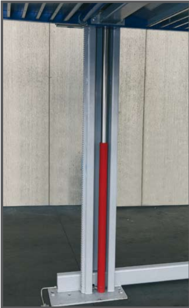
The hydraulic double extension lifting cylinders (RAM - manufactured by O.M.E.R. S.p.A.) permits direct lifting, without any auxiliary aids such as cables or chains.
