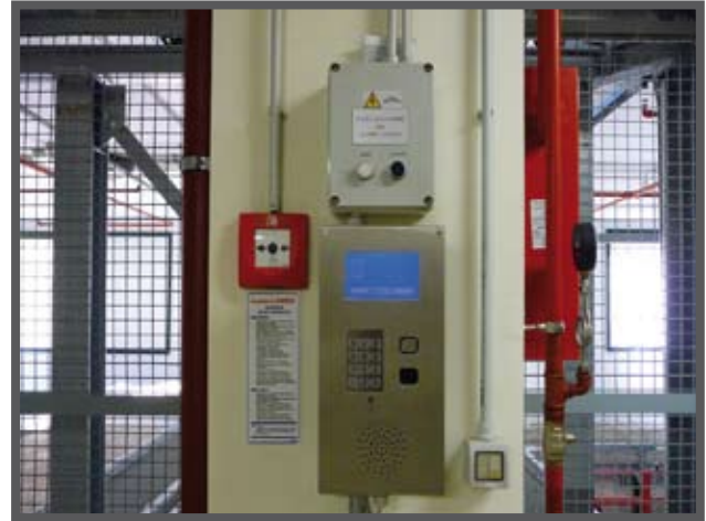
Fig 5: Detail of the operator panel used to provide information and to enter the access codes for parking and picking up vehicles.
