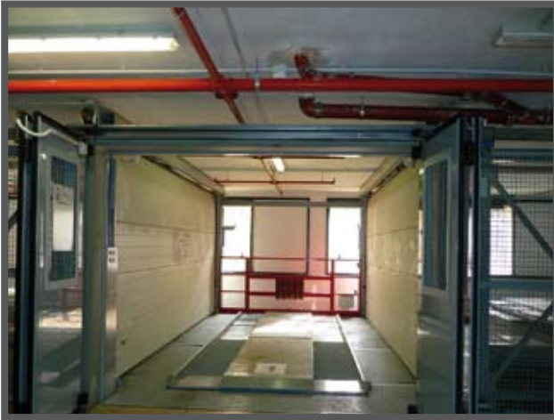
Fig 1: Vehicle entrance to control positioning on platform. Entrance is protected from the vehicle storage zone by two sectional doors.
