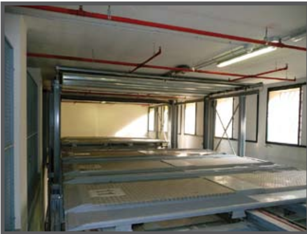
Fig 2: Area beside the entrance where the vehicle platforms are stored.
